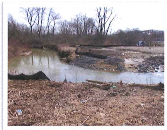
The photo above shows the improper installation of stormwater management controls for new construction. Act 167 Stormwater Management Plans, and associated ordinances require proper management of stormwater runoff from new development and redevelopment projects.
